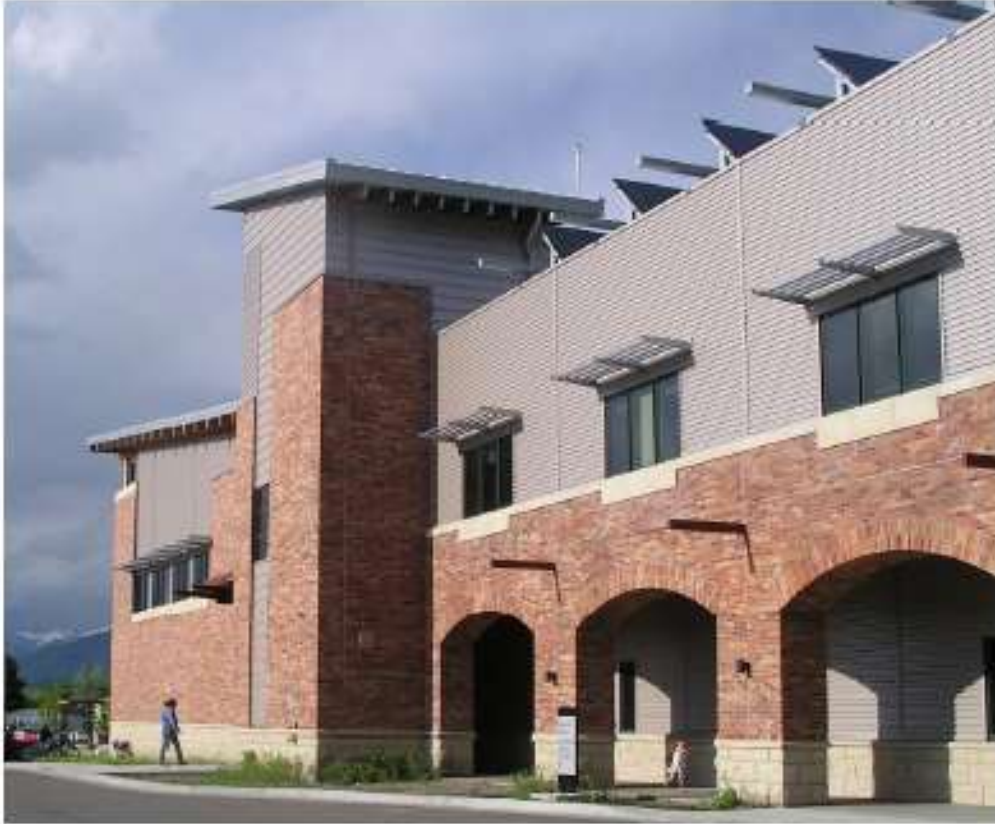
Figure 4-33. Articulation, Materials, and Design of Side and Rear Facades
