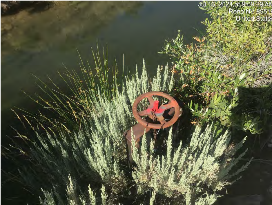
Photograph 33: Water main/gate. Note, no water was flowing out. Image 4370 Date: July 16, 2021
