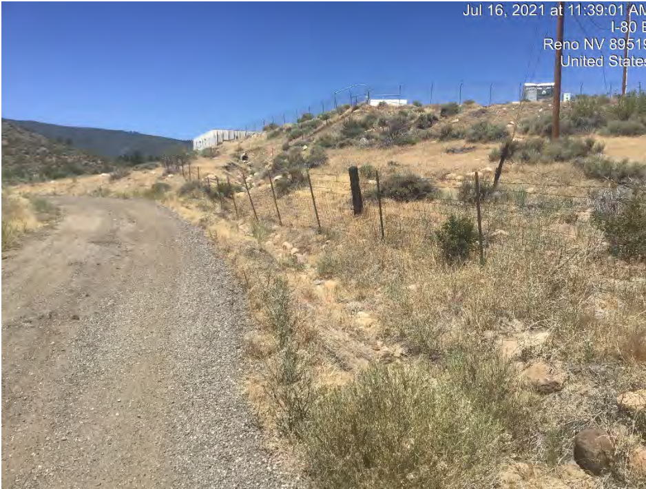
Photograph 103: Draining next to NF-100 Road. Utility(?) buildings in the background. Photo facing northwest. Image 4447 Date: July 16, 2021
