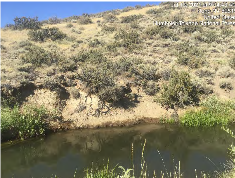
Photograph 32: Steamboat Ditch with seeps along dirt impoundment. Photo facing south. Image 4369 Date: July 16, 2021
