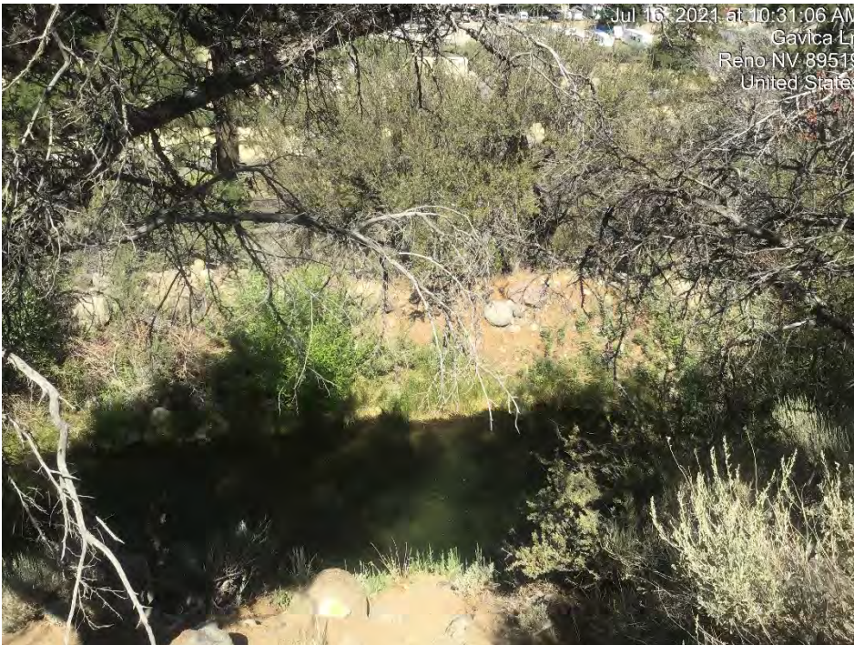
Photograph 78: Steamboat Ditch with dirt embankment. Photo facing the ditch.
