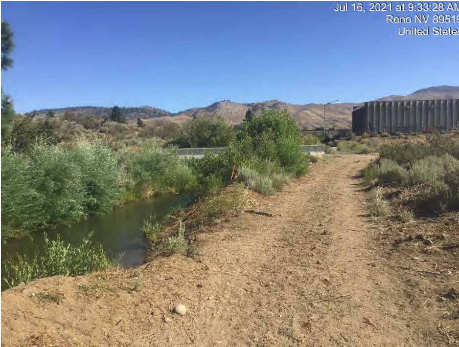
Photograph 51: Steamboat Ditch Trail, concrete bridge crossing. Photo facing north.
