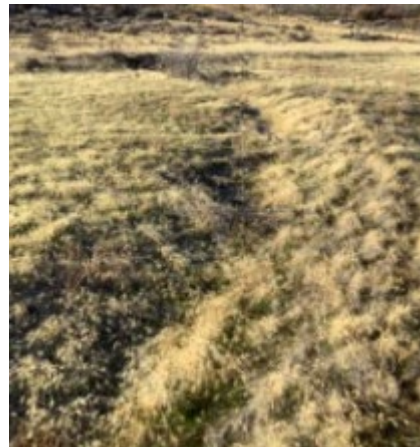
Photograph 20: Minor ditches carry stormwater under Boomtown-Garson Road from Steamboat Ditch to the stormwater swale area; facing south. Note culvert at top of photo for road crossing (Image 0344)
