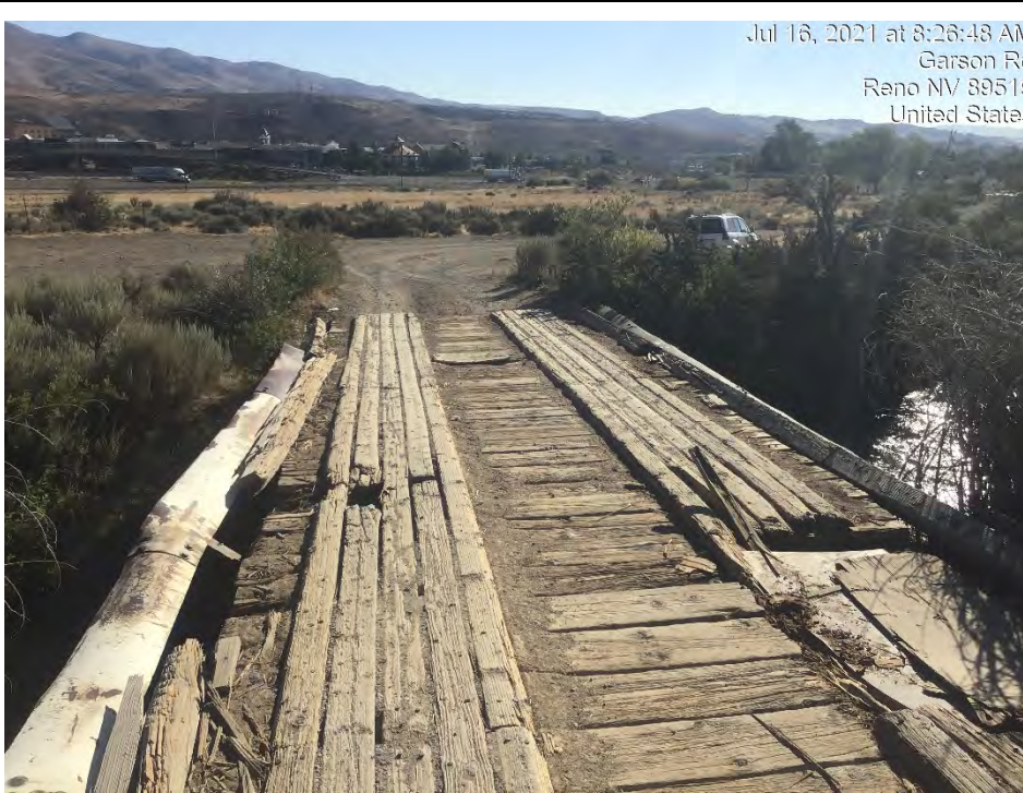
Photograph 1: NF-100 Road bridge crossing. Photo facing north/northeast. Image 4336 Date: July 16, 2021
