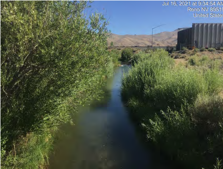
Photograph 53: Steamboat Ditch from the concrete bridge. Photo facing north. Image 4392 Date: July 16, 2021
