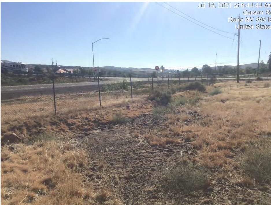
Photograph 20: Drainage area near fence between gravel road and Highway 80 East. Photo facing east. Image 4356 Date: July 16, 2021
