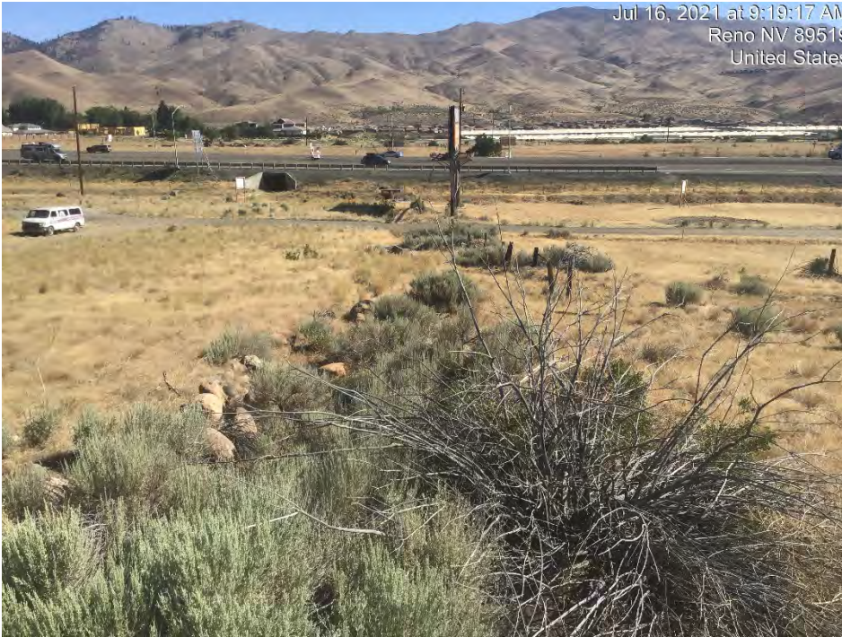
Photograph 41: Rock lined drainage from Steamboat Ditch. Photo facing north. Image 4379 Date: July 16, 2021
