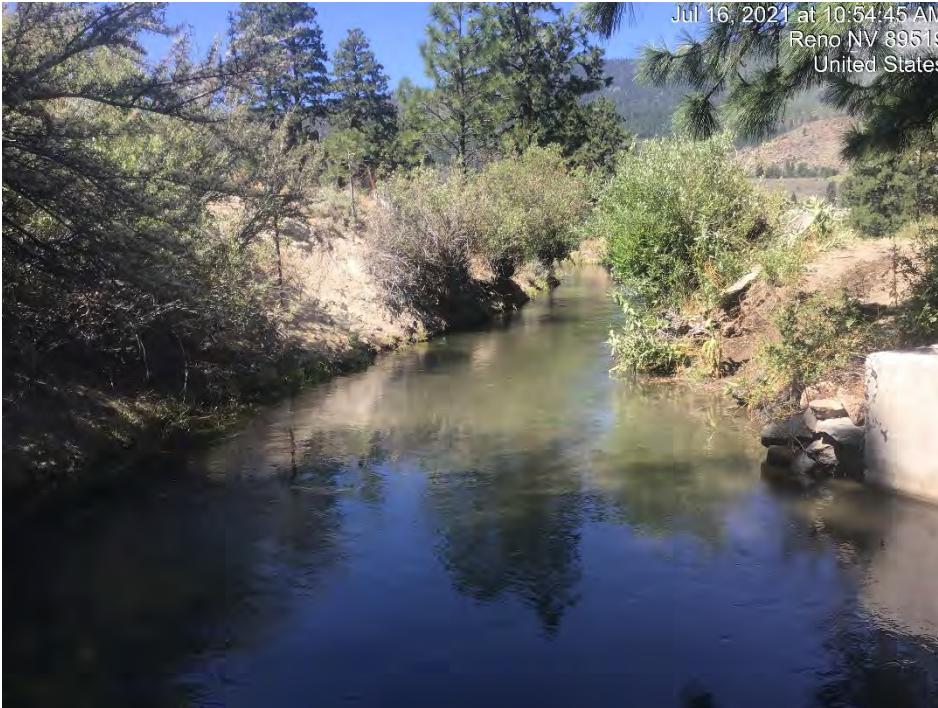
Photograph 99: Culvert with flashboards at the Steamboat Ditch and drainage intersection. Photo facing west. Image 4442 Date: July 16, 2021
