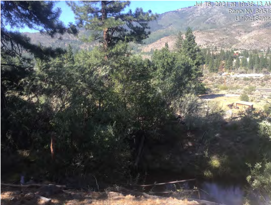
Photograph 85: Steamboat Ditch with gate. Photo facing west.
