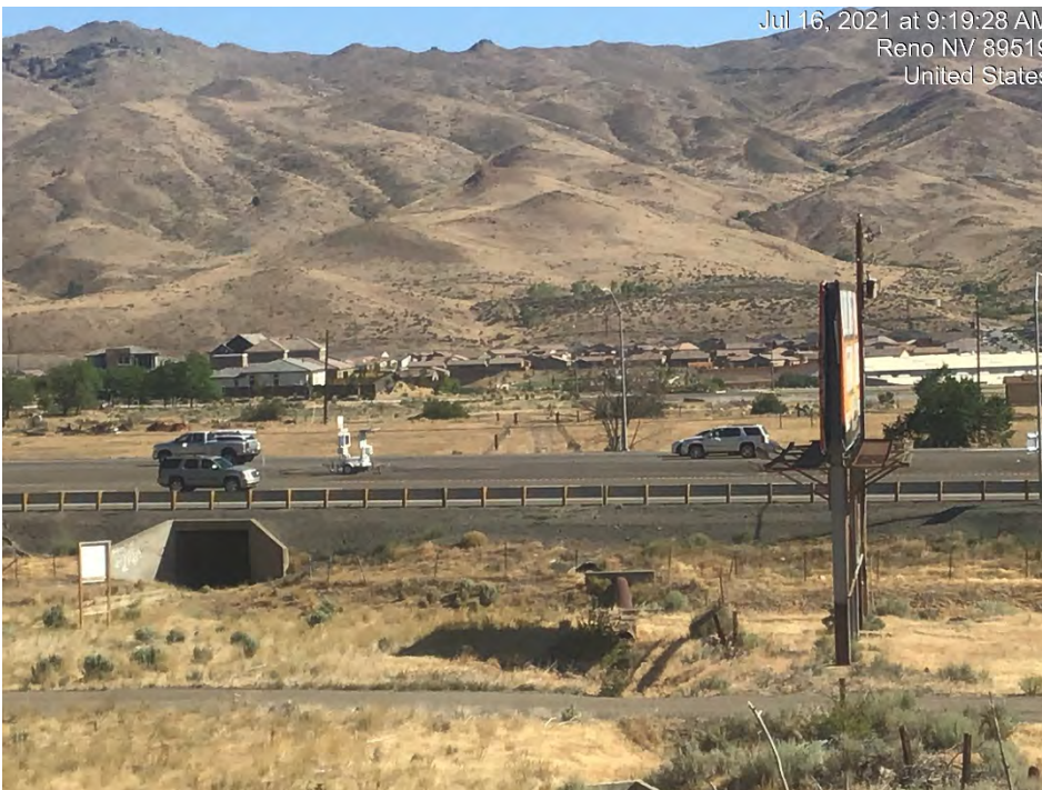
Photograph 42: Rock lined drainage intersection to drainage area that flows under Highway 80 from Steamboat Ditch. Photo facing north. Image 4381 Date: July 16, 2021
