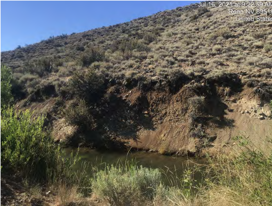
Photograph 43: Dirt banks of Steamboat Ditch. Photo facing south. Image 4382 Date: July 16, 2021
