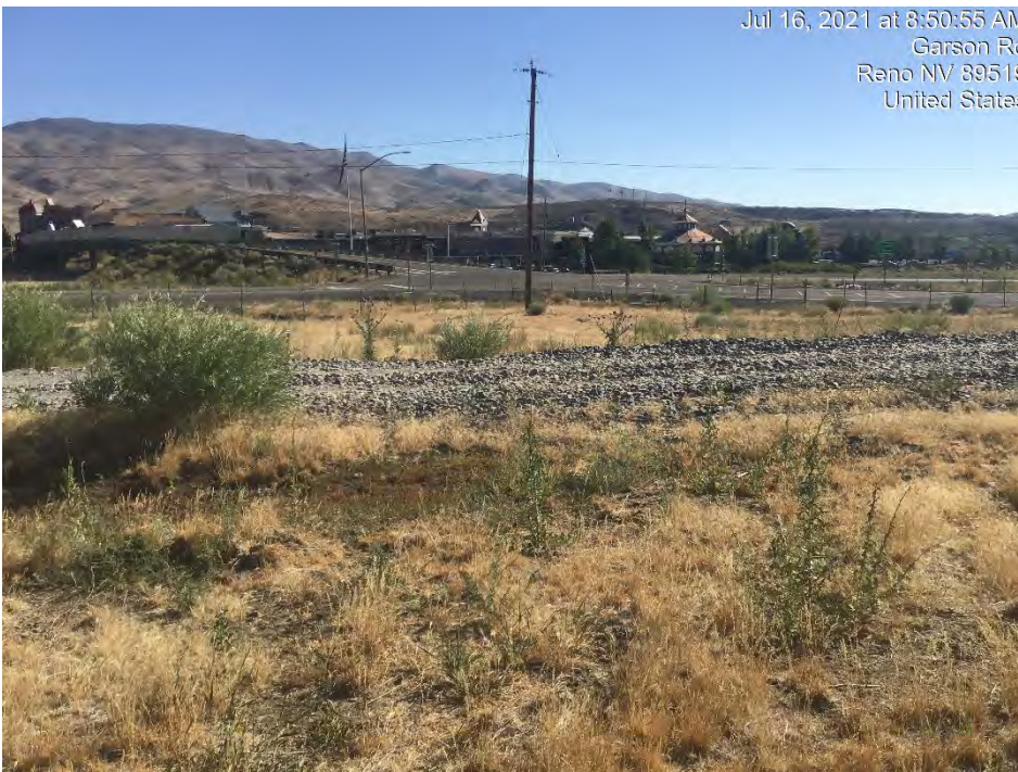
Photograph 26: Low point off gravel road which has washed out and been repaired with coarse road gravels. Photo facing north.
