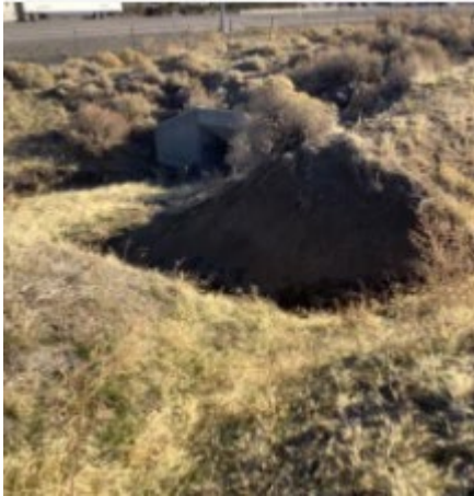
Photograph 21: Stormwater swale flows into 48" RCB at east end of swale close to corner of Cabelas Store building; facing northeast (Image 0294)
