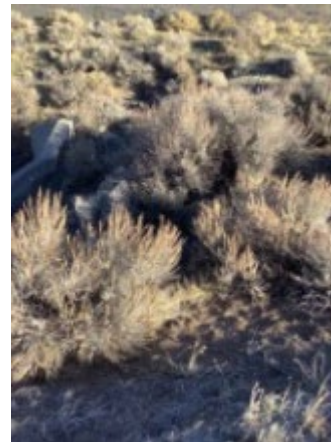
Photograph 22: Native vegetation over storm drain box culvert as water heads east; facing north (Image 0295)
