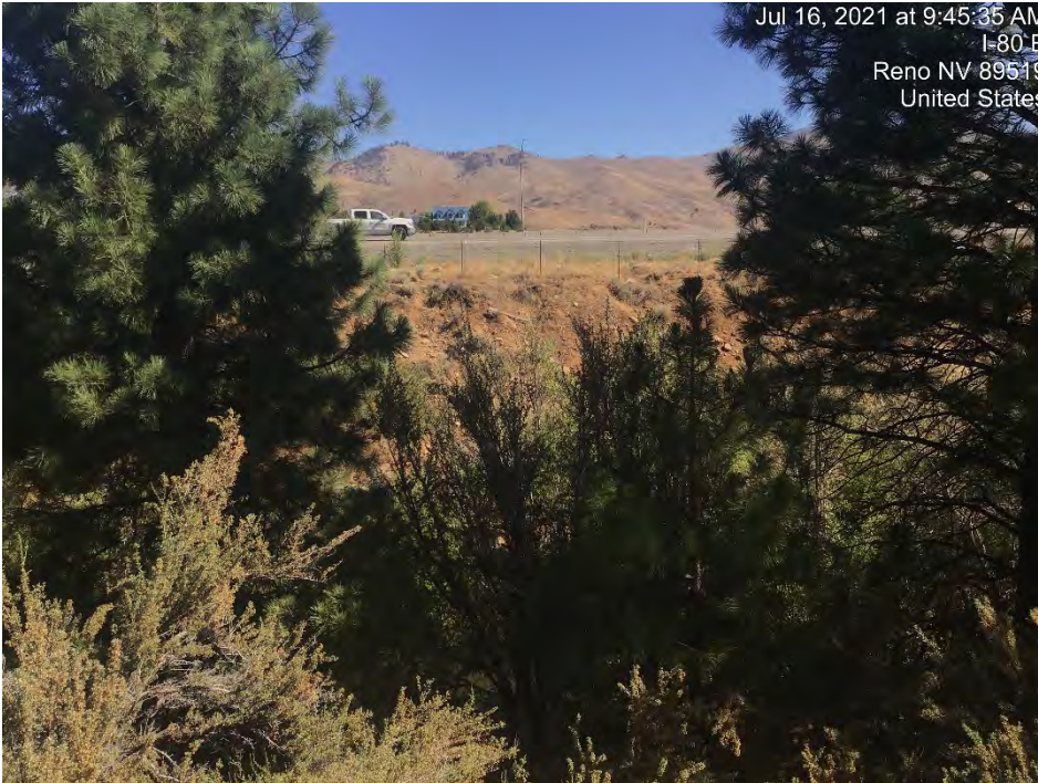
Photograph 55: Dirt embankment incised on ditch. Photo facing north/northwest. Image 4394 Date: July 16, 2021
