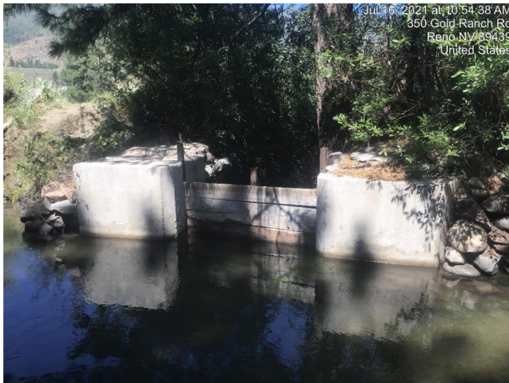
Figure 1: Existing Flashboard Gate located above Channel-2 at the Steamboat Ditch.
