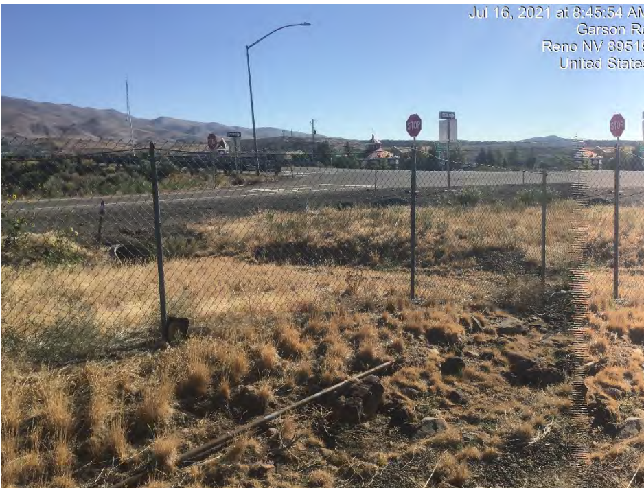
Photograph 24: Drainage area near gravel road. Photo facing east/northeast.
