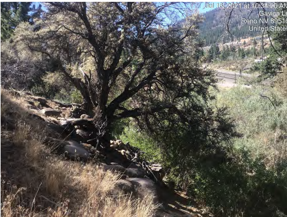
Photograph 82: Steamboat Ditch with heavy vegetation. Photo facing west. Image 4422 Date: July 16, 2021
