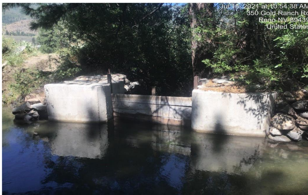
Figure 1: Existing Flashboard Gate located above Channel-2 at the Steamboat Ditch.
