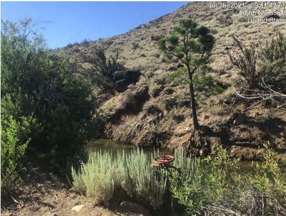
Photograph 34: Water main/gate. Note, no water was flowing out. Photo facing south. Image 4371 Date: July 16, 2021
