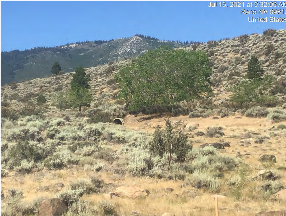
Photograph 49: Drainage pipe above Steamboat Ditch in the background, zoomed in. Photo facing south.
