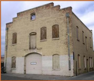
example of construction methods for that period. In 1936, a rear addition was added using the same design and material elements. The building contains a total of 3,268 sq. ft. and is built of solid brick walls with truss floor construction. It was constructed in the Mission/Spanish Revival elements similar to railroad depot designs which
